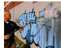
Rinsing larger graffiti after applying BBSM
